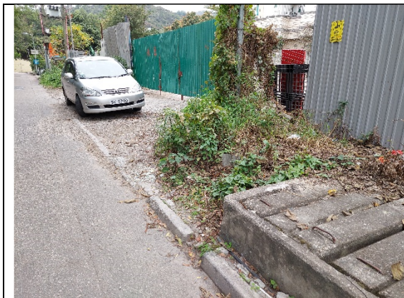
Plate No. 3 – Existing conditions of the subject site entrance (Existing Catchpit 1 is located on the right hand side of the entrance but no existing 450U channel is found)
